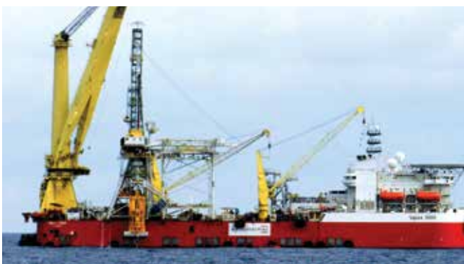
Installation of SLED using the J-Lay tower.
